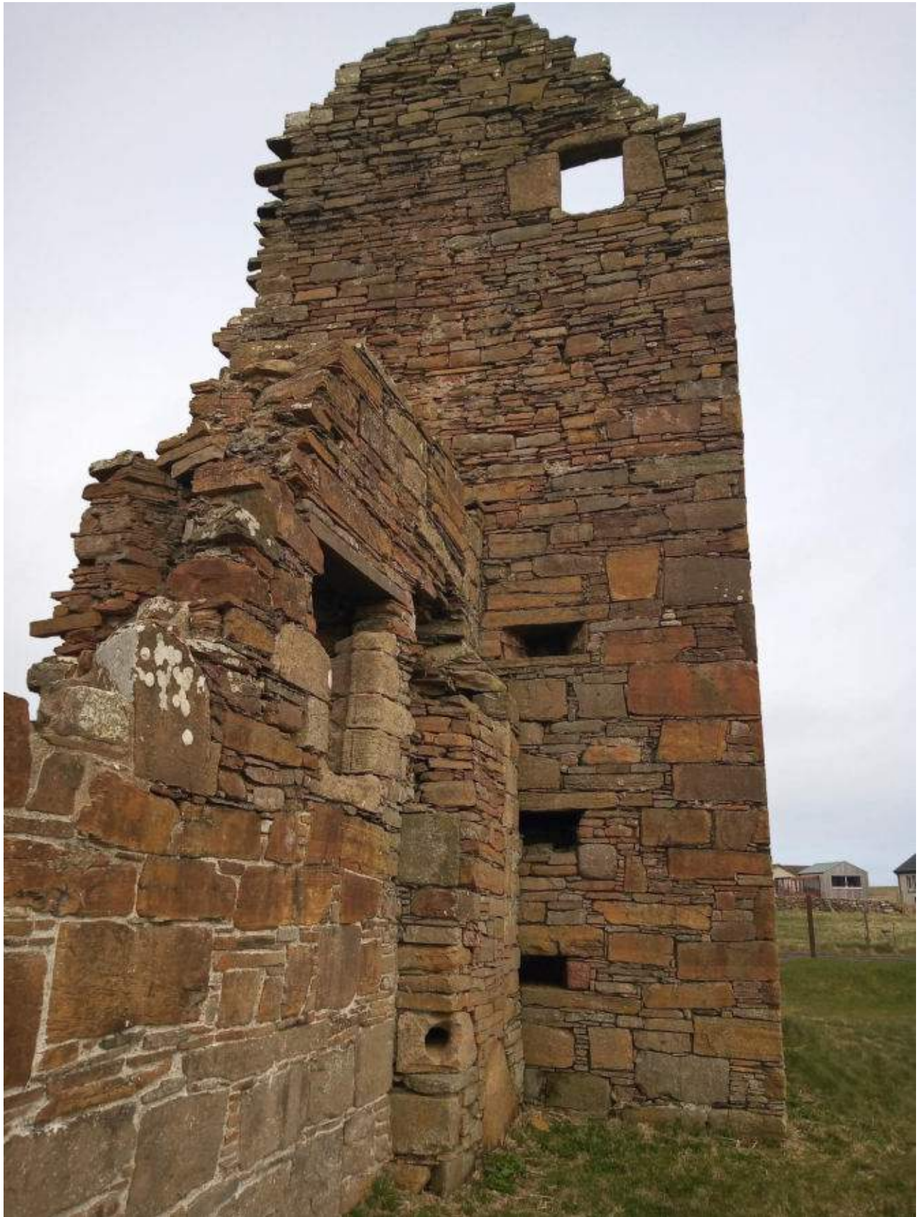
Plate 24: View north of Earl's Palace HES PiC (Asset 123) northeast corner tower
