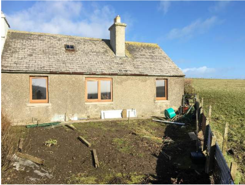
Photographs of SLM in position & identified noise sources
